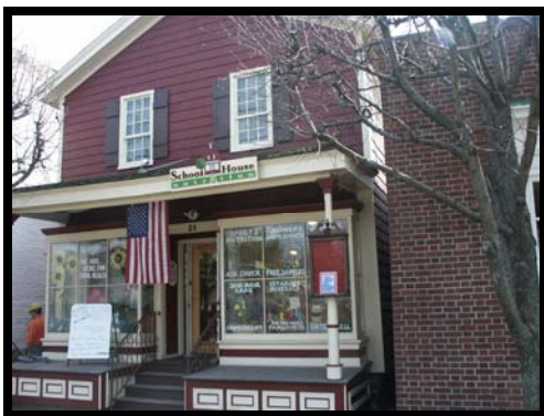
Protected Town Landmark, Little Red Schoolhouse, 21 Tokeneke Road. (Darien's oldest public building)
